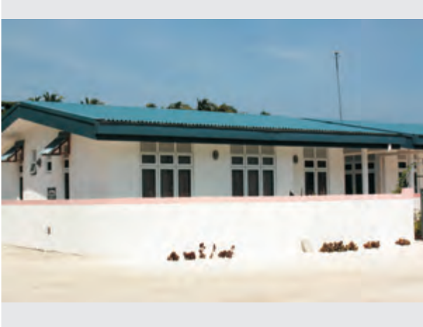
Figure 6.14: Government sponsored houses constructed for migrant communities from Faridhoo, Kunburudhoo and Maavaidhoo on the Island of Nolhivaranfaru. Houses were allotted to families by chance when two students from the “host” island drew lots to determine which house would be allocated to which family. This allotment procedure was seen as a “fair and good process”. (Q18/Migr/Dest/Nolhivaranfaru/20111229).
