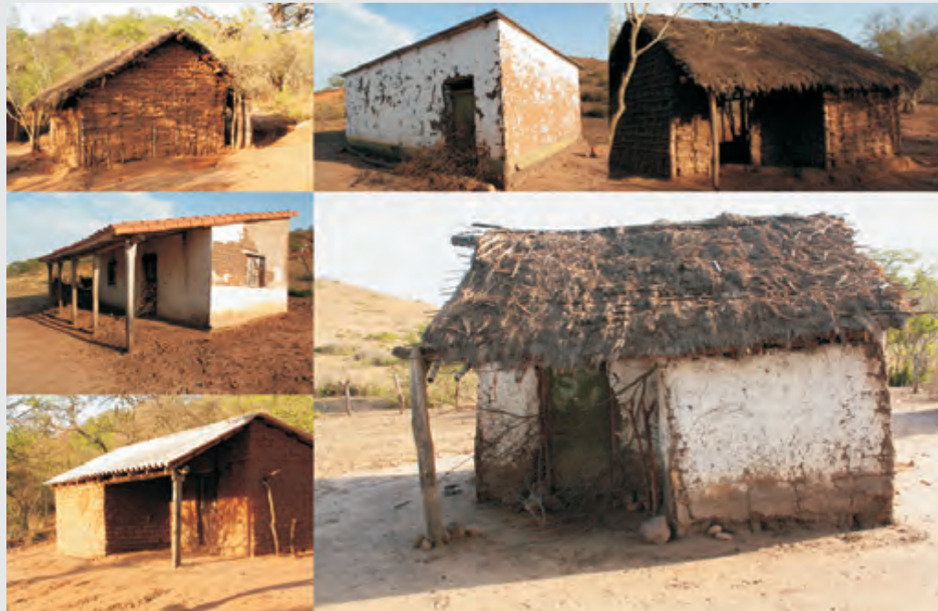
Figure 4.4: Abandoned houses in out-migration affected Guaraní communities visited during field research in Bolivia's Gran Chaco (Photo: Johannes Luetz, December 2010)
