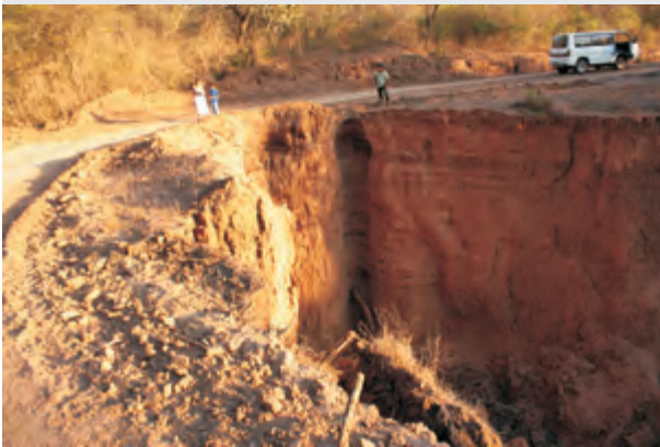
Figure 4.25: Erosion along the route from Camiri to Charagua in the vicinity of Caipipendi, 18 December 2010. (Photo: Johannes Luetz)
