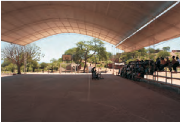
Figure 4.20: Elaborate multipurpose rain catchment system. The enormous roof size of this basketball and football field provides shade for sports activities and community meetings (ongoing, right), as well as a significant catchment area to funnel rain water into an adjacent tank (see Figure 4.21). (Photo: Johannes Luetz, 16.12.2010)
