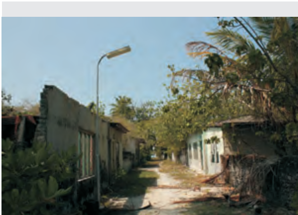
Figure 6.7: On 5 July 2007 the Maldivian government moved the entire community of Hathifushi Island (“community of origin”) to settle on Hanimaadhoo Island (“community of destination”). With the exception of three temporary resident caretakers Hathifushi is now classified as “uninhabited”. Affected respondents indicated that they are still waiting for new houses in Hanimaadhoo, expressing disappointment at the slow resettlement process. (Hathifushi Island, Q27/Orig/Hathifushi/20111231).
