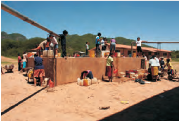
Figure 4.21: This tank collects water from the adjacent roofed-over basketball court (see Figure 4.20). The popularity of this rain catchment system was apparent on the day of the research visit to the community, with dozens of children carting away buckets of water. The locked tank is only opened for two hours in the morning Tuesdays, Thursdays and Saturdays. (Carlos Lazarte; Q13/Exp/Orig/EI Cruce/20101215; Photo: Johannes Luetz, 16.12.2010)
